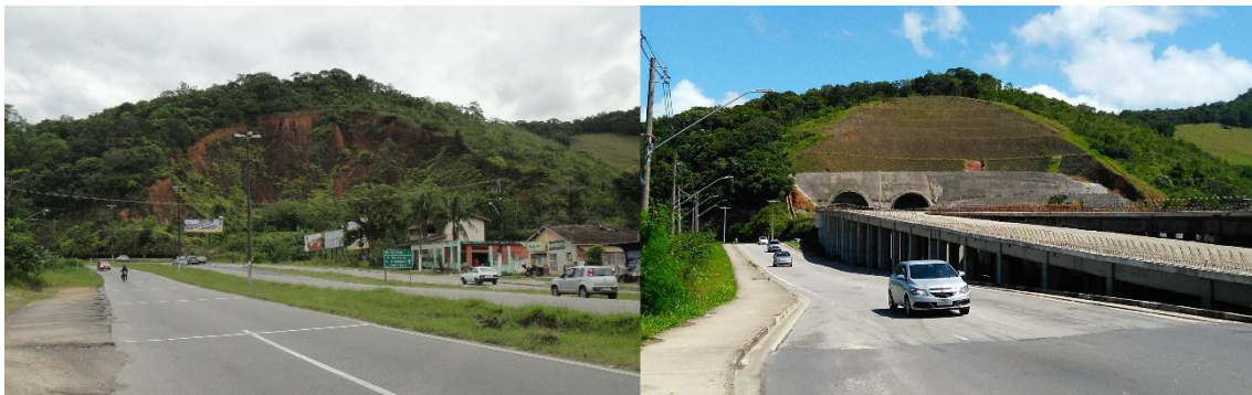
Figure 6. T101 northern portal before (left) and after (right) construction and erosion control measures.
