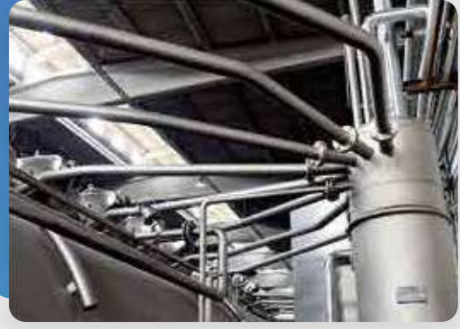
DÜZE TRANSFER BORULARI NOZZLE TRANSFER PIPES
