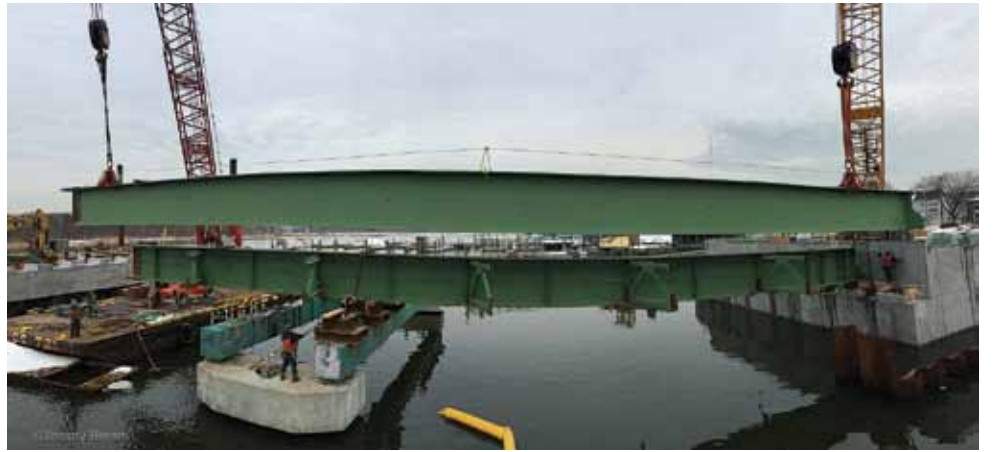
Photos by JAMES BREEN and ANGELO BELLOCHIO The contractor has been installing steel stringers on the piers of the new bridge in preparation for the deck construction and building the abutment on the Park side of the bridge. The Department of Transportation estimates that work will be completed during the summer. Check on the project progress by visiting the Facebook page City Island Bridge or by contacting the DOT liaison, Huascar Robles, at cityislandbridgehbx1164@gmail.com . The Bronx Boy Scouts patch has also undergone a redesign, now honoring the old City Island bridge (below).
