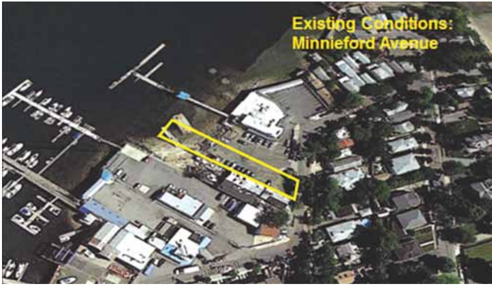
Photos courtesy of NYC DEPARTMENT OF DESIGN AND CONSTRUCTION
