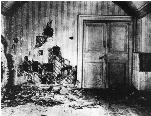
THE ROOM IN IPATIEV HOUSE WHERE THE ROMANOV ROYALS WERE MURDERED.
