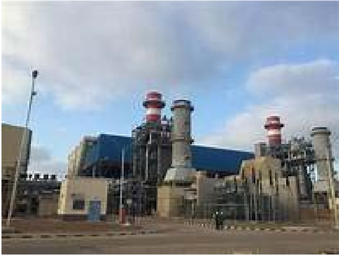
Project Name: Damietta Combined Cycle Power Plant Client : Egyptrol Scope of work : Design of DCS Tender Package
