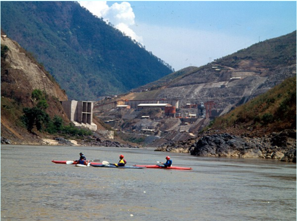
Huge intakes are on left.
