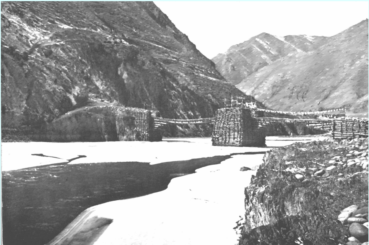
Old bridge in winter picture.
