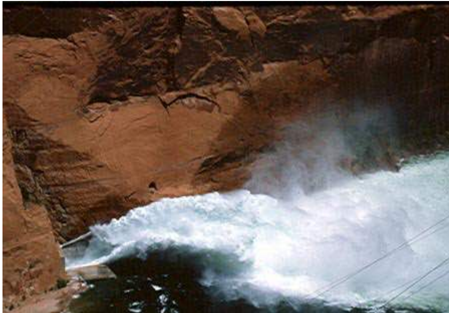
The left spillway at Glen Canyon Dam, 1983. The right spill way was closed due to fear of damage from harmonic vibrations.
