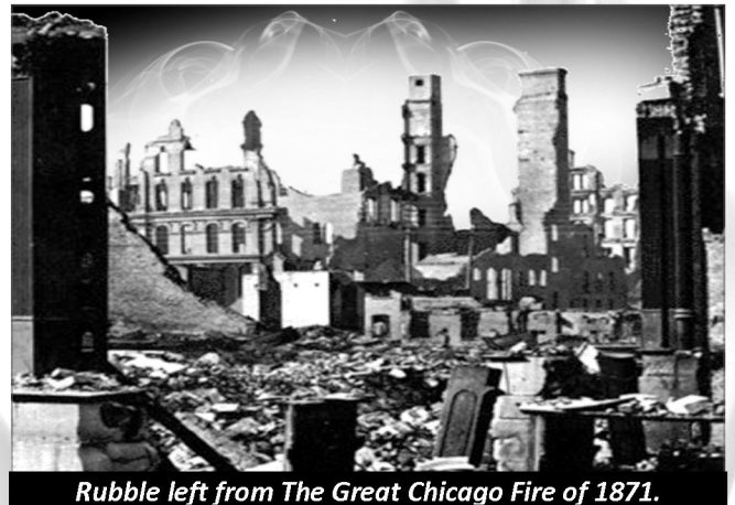
Rubble left from The Great Chicago Fire of 1871.
