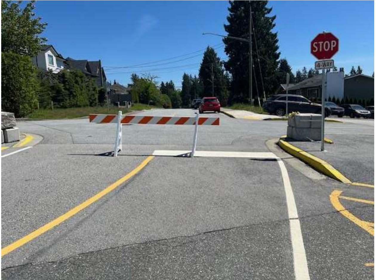
This is the barrier that keeps vehicles from driving into the road space the children use to get to the current play areas.
