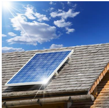
Solar panel on the roof
