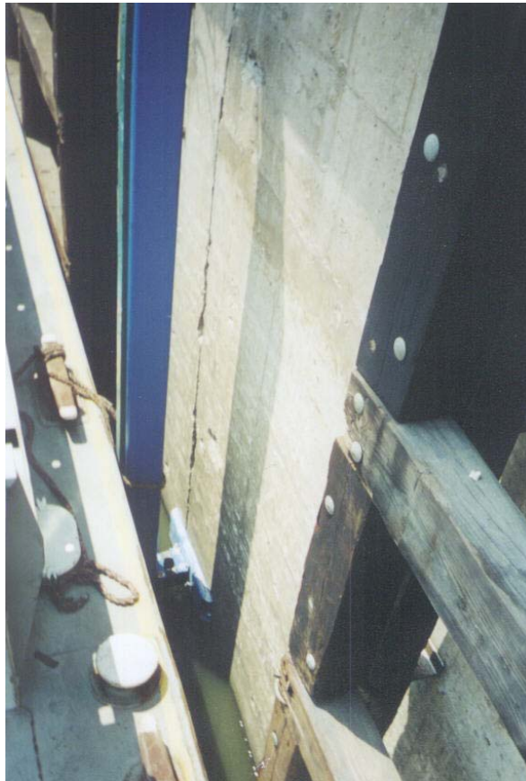
DOCK-SHOCK Model DS10-20V Port of Catoosa, Oklahoma 10-Units Anchored to Concrete Wall Used for cushioning and mooring, allowing for 20 Feet water level fluctuation.
