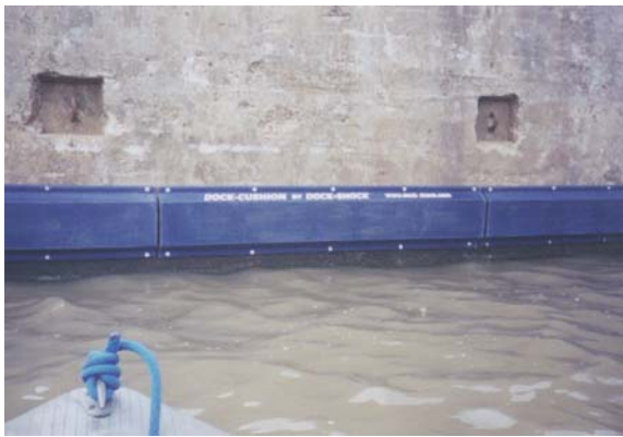
DOCK-CUSHION By DOCK-SHOCK Port of Catoosa, OK - Low Water Dock 25 – Units Anchored to Concrete
