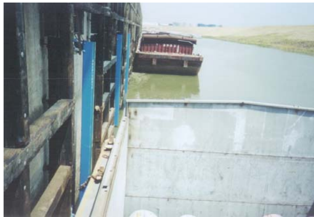
DOCK-SHOCK Model DS10-20V Port of Catoosa, Oklahoma 10-Units Anchored to Concrete Wall Used for cushioning and mooring, allowing for 20 Feet water level fluctuation.
