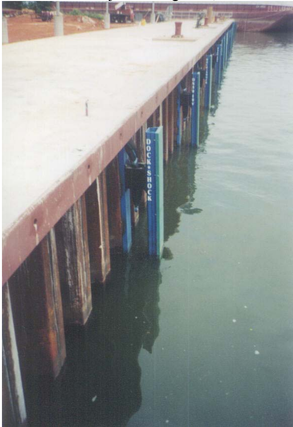
DOCK-SHOCK Model DS50-10V Port of Decatur, Alabama Roll On–Roll Off. Dock used for the loading of the Boeing Delta IV Rocket. The installation used 25 - units welded to steel sheet piling Total Project Savings $25,000.
