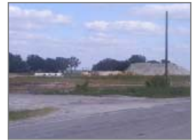
Construction site off Fruitville Road
