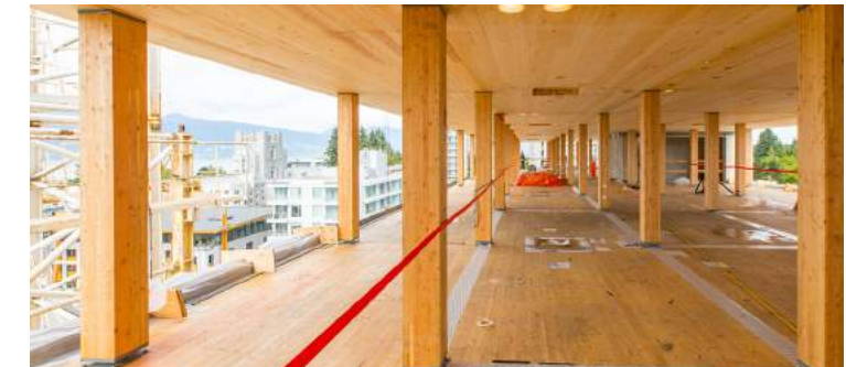
UBC's Brock Commons Tallwood Student House —the world's tallest contemporary wooden building at 18 storeys (54 metres/approx 177 feet)—showcases the advantages of building with wood.
