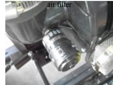
Dry-type air filter blockage alarm
