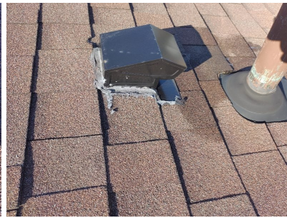
Excess sealant around roof vent.
