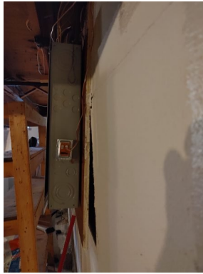
Electrical panel has separated from the foundation.
