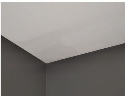
Discoloration of the ceiling in the rear right corner.
