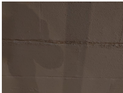
Horizontal crack.
