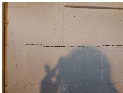
Second Horizontal Crack
