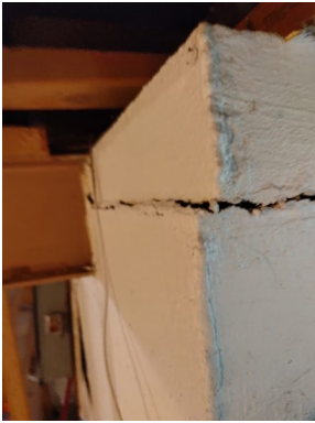
Open joint. The block have begun to slip off of each other.
