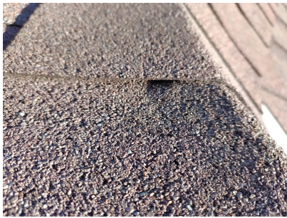
Raising shingle which could allow water to penetrate.
