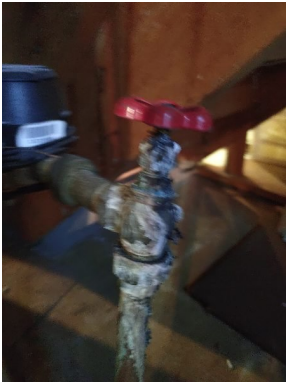
Corrosion around the water entrance and main shutoff valve.
