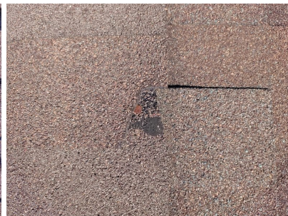
Exposed, rusted nail.
