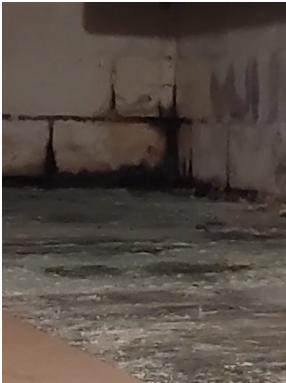
Signs of water penetration within the crawl space. This is the same area as the step cracks in the outside brick.
