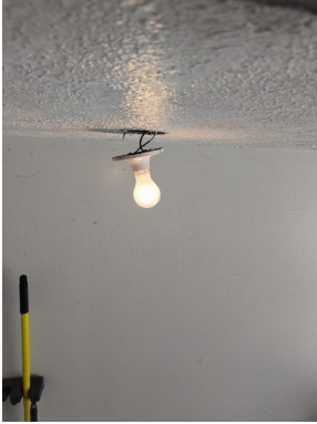
light is not properly attached
