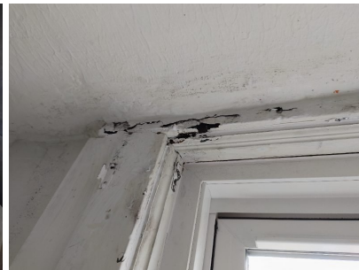
Wood has begun to deteriorate around the attic window.
