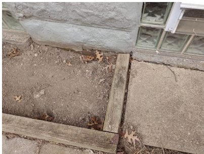
Low section in the rear of the home where water can pool against the foundation.
