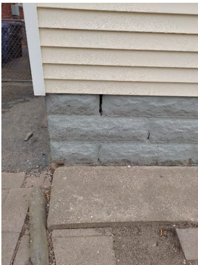
Mortar missing from foundation
