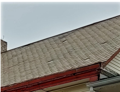
Missing Singles and Some Raised Shingles. Recommend further evaluation by a licensed contractor.
