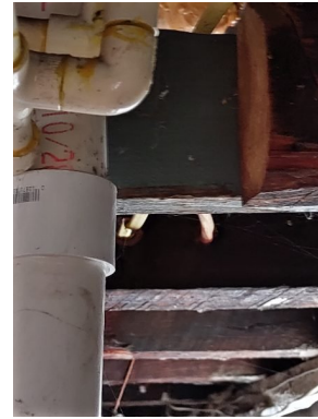
Missing section of the floor joist.
