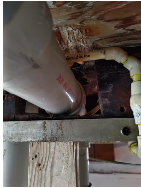
Notched floor joist with wood post re-supporting the joist.
