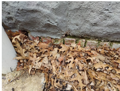
Foundation is not properly sealed, allowing water to penetrate.
