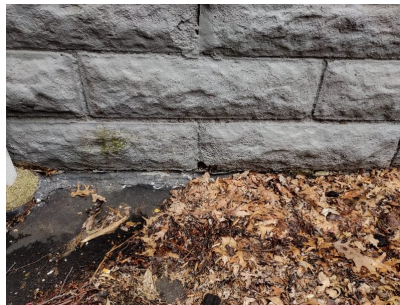
Slight pitch toward the home on the driveway side of the home.
