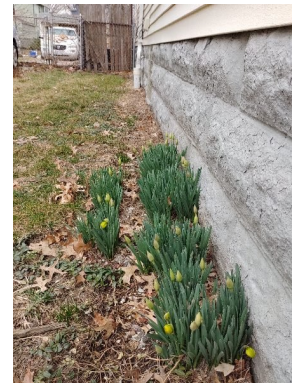
Low areas along the non driveway side of then home where water to pool and rest against the foundation.
