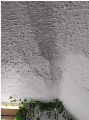
Attic ceiling is uneven.
