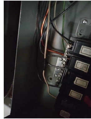
Improper splice
