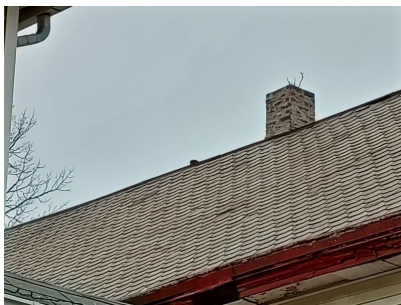
Stick protruding from the chimney.
