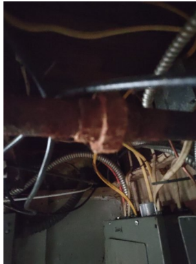
Gas line union shows signs of rust and sits above the electrical panels.
