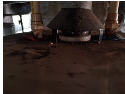
Build up around the Hot Water out and Cold Water In.
