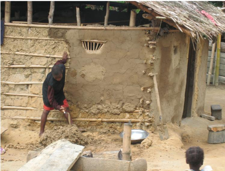
**STUCCOING THE OUTSIDE.** Dirt is mixed with cement powder and the surface that results is pretty much impervious to rain.
