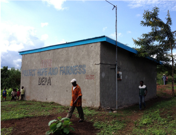
Rice Hulling Building
