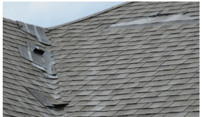
Missing Shingles
