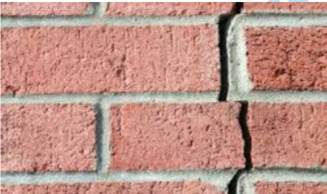
Cracking in the bricks at the back of the house
