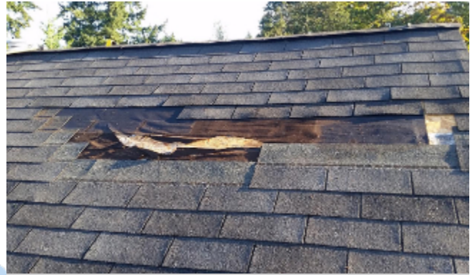
Missing Shingles
