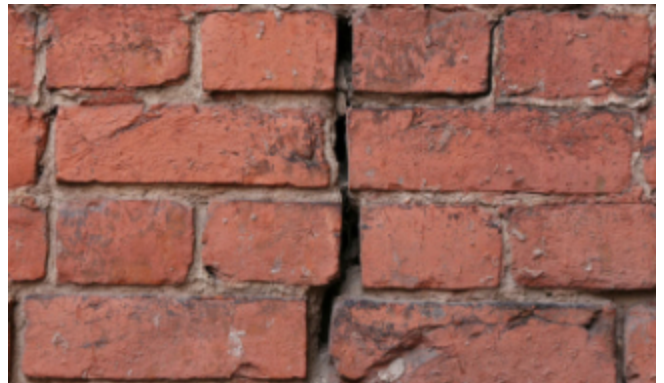
Cracking in the bricks on the north side of the house
