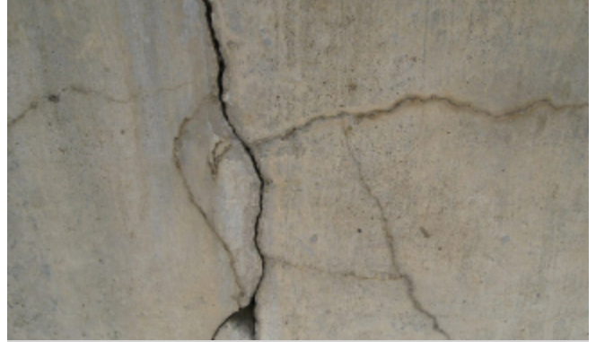
The foundation itself is cracked
