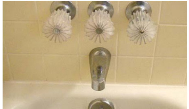
Tub, tile and plumbing fixtures are all original from 1950s.
