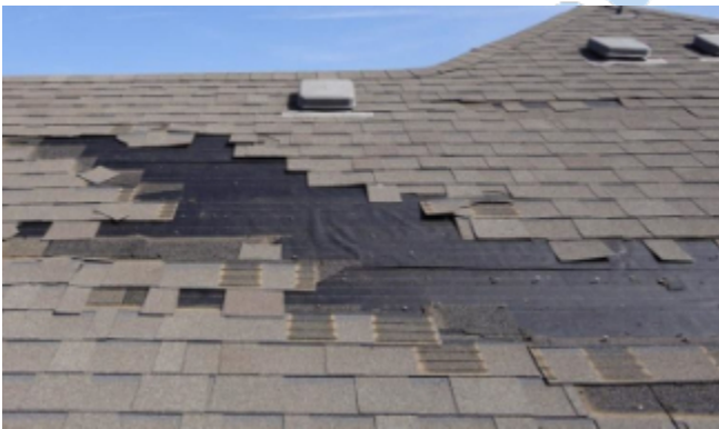
Missing Shingles
