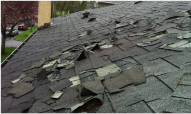
Missing Shingles
