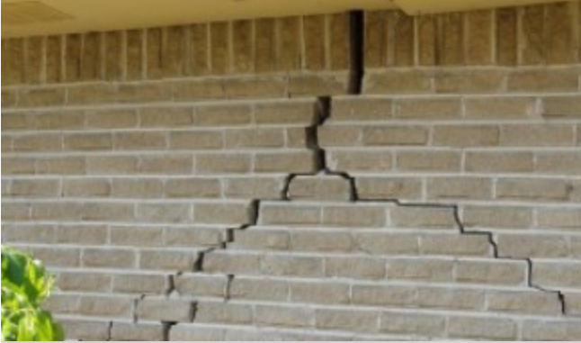
Major cracks on the south side of the house
