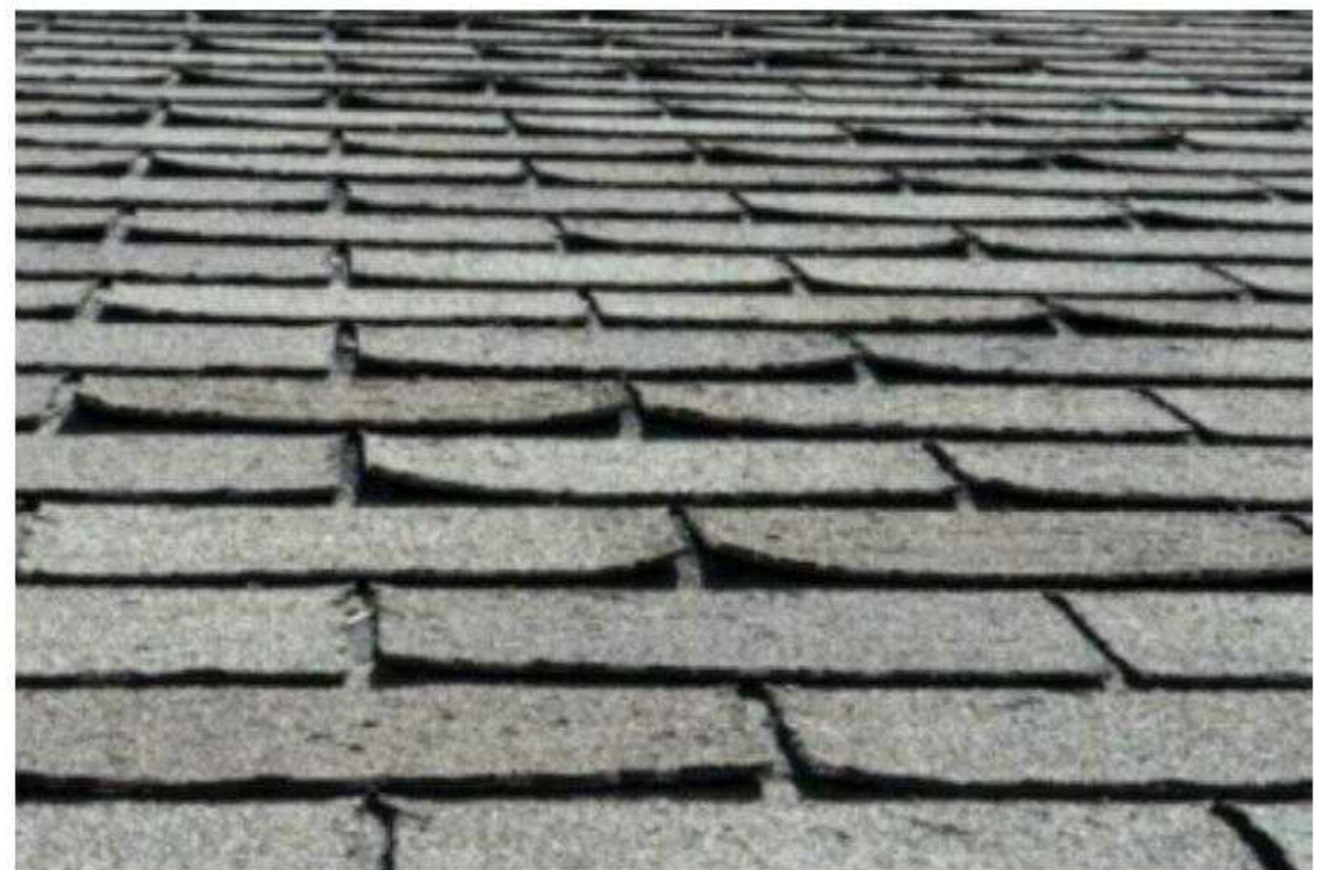
Tile are starting to curl up in multiple locations.
