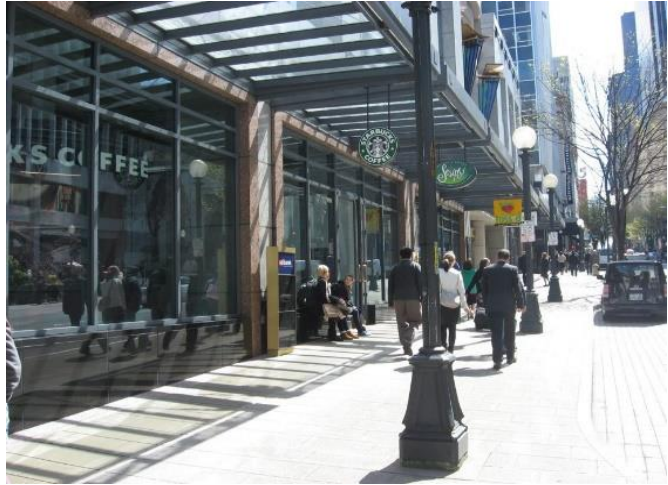
Figure 7.26 - Awnings over sidewalk in Seattle, photo by nacto.org
