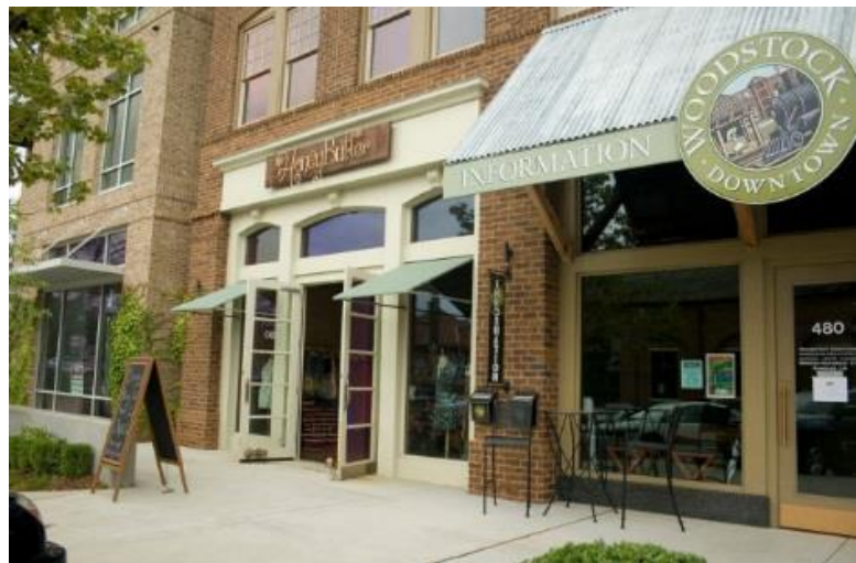
Figure 7.24 - Facades with Windows and Doors
