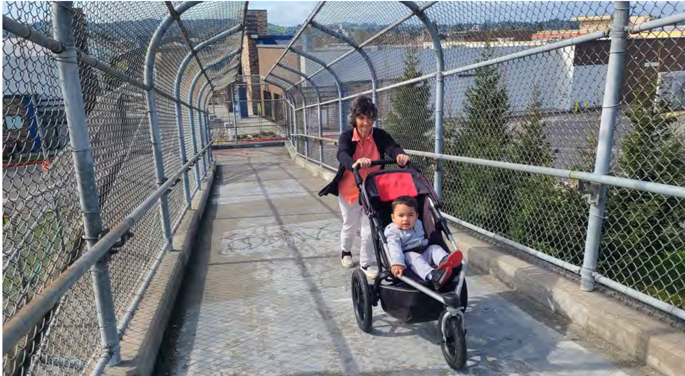
View West on McKenzie Overcrossing
