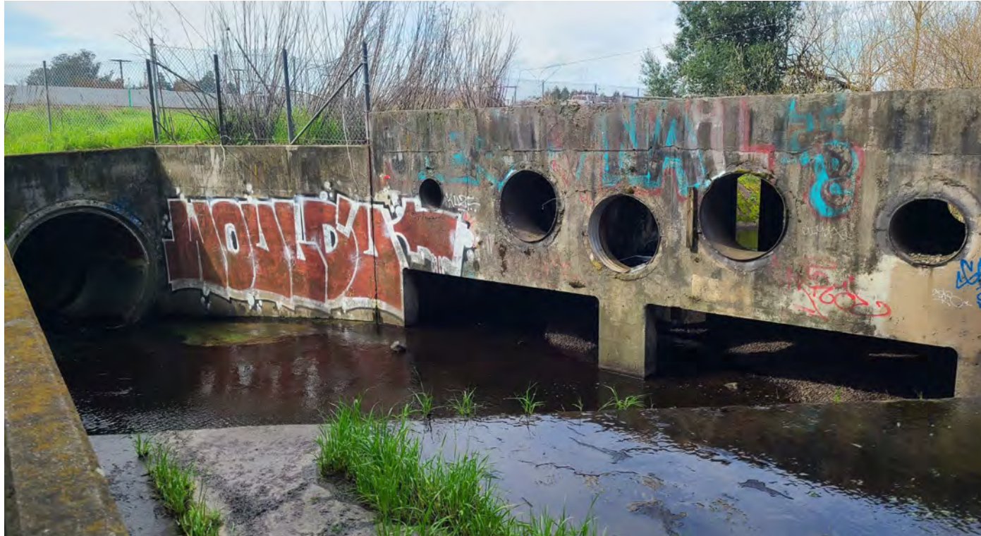
View of Drainage Structure on North Side of Corona Rd
