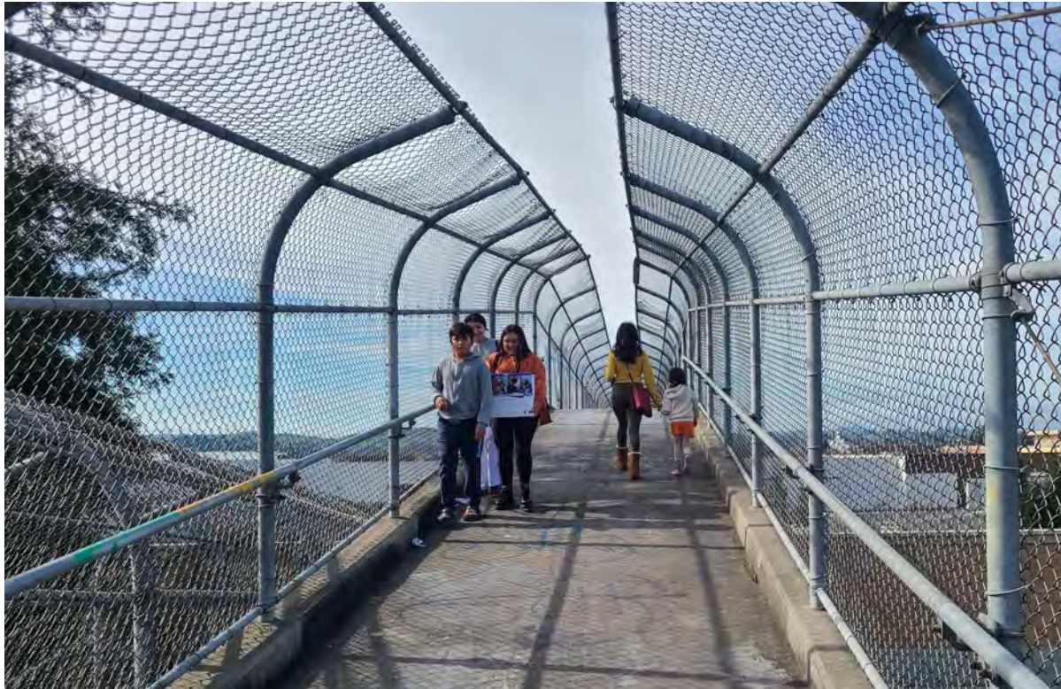
View West on McKenzie Overcrossing
