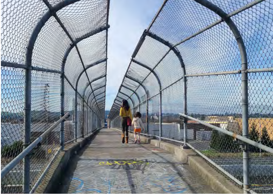
2" Openings (Existing Structure)
