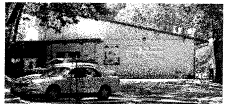
The 50-year old facility needs major renovations.
