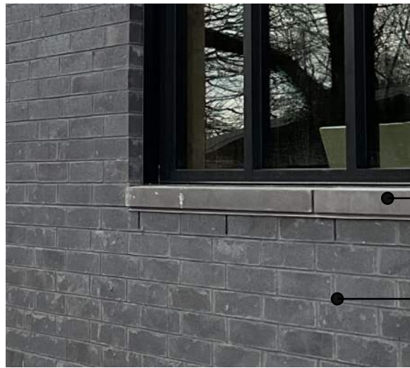
IMAGE OF BUILDING FOR REFERENCE
