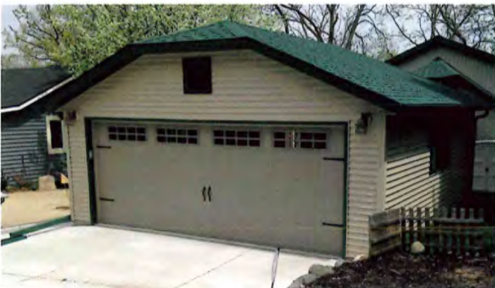
This clipped gable garage perfectly matches the roof style of this home.
