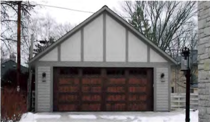
This Wauwatosa garage adds to the charm of the house. The custom overhead door brings out the features of the house.
