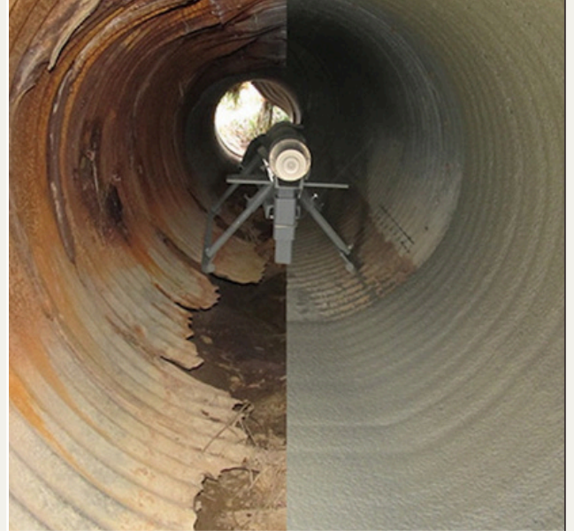
Sanitary Sewer Rehabilitation Project
