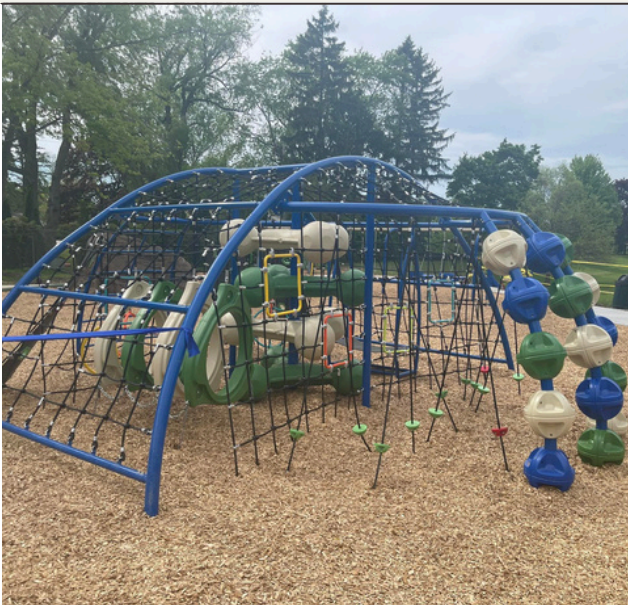
Ellsworth Park Playground Renovation
