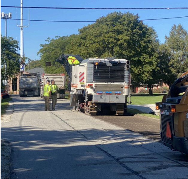
Road Resurfacing and Stormwater Project
