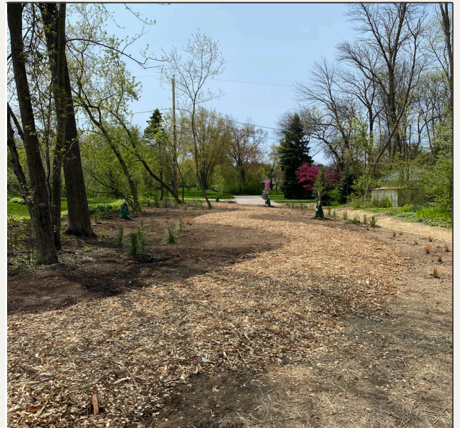
Tennyson Trail Rehabilitation
