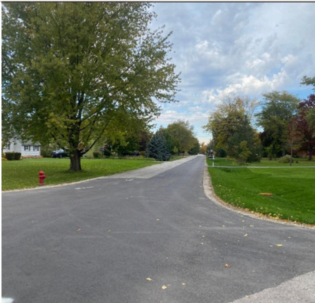
East Bayside Sanitary Sewer Relief System
