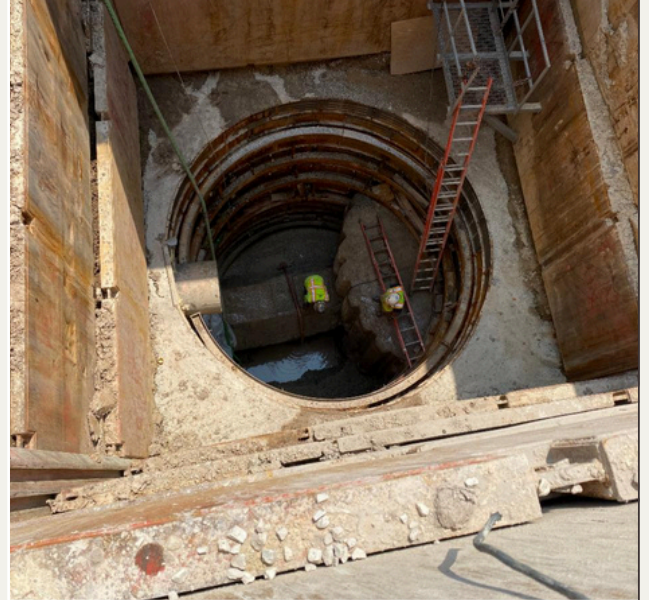
Brown Deer Road Sanitary Sewer Replacement
