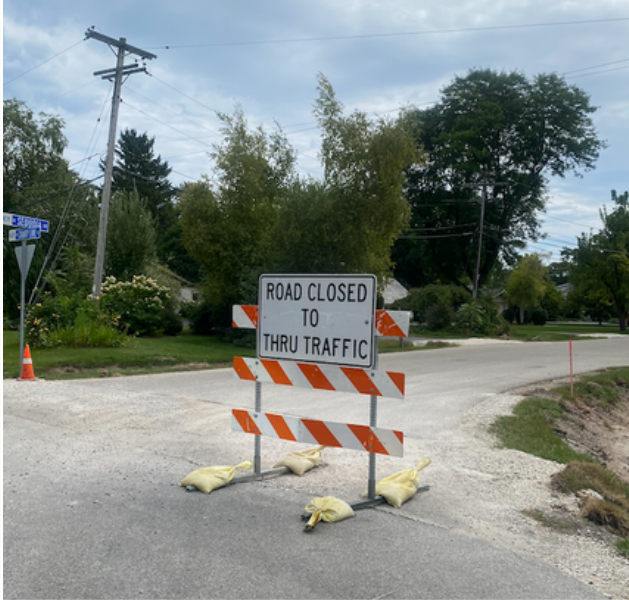
Road Resurfacing and Stormwater Project
