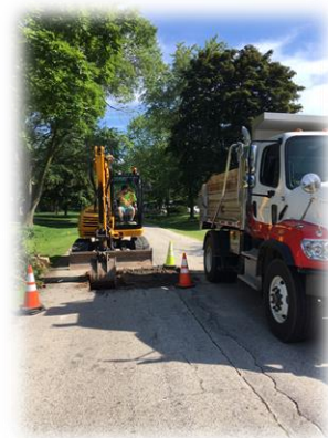
DPW Manhole Rehabilitation
