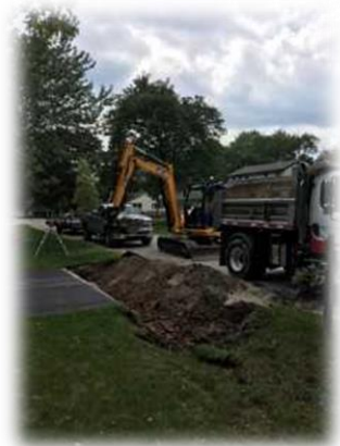
Culvert Pipe Installation
