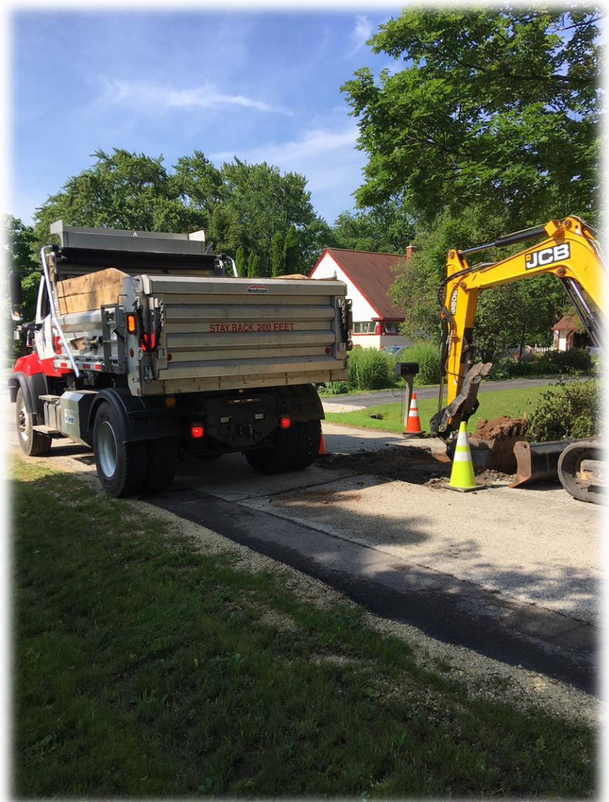
Public Works Manhole Rehabilitation
