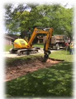
Ditch Re-Grading
