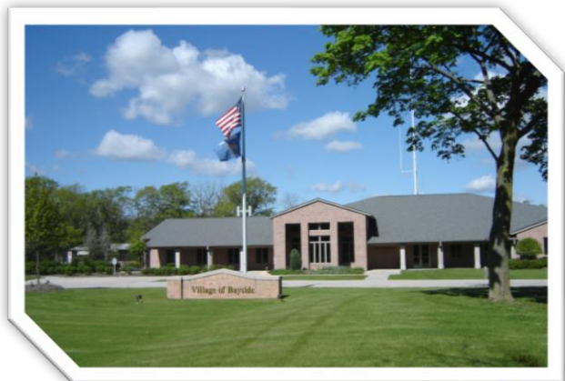
Bayside Village Hall
