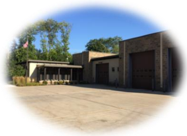
North Shore Fire/Rescue Station #85
