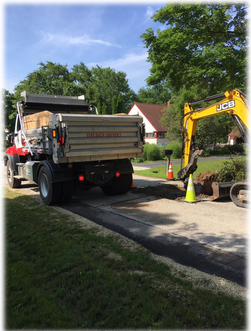
Public Works Manhole Rehabilitation
