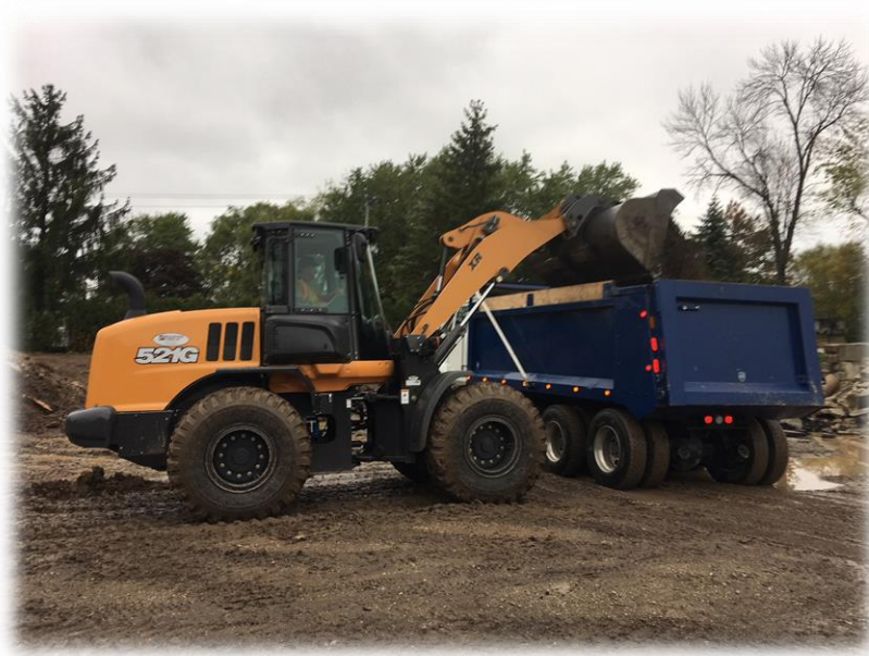
Public Works Yard Clean-up
