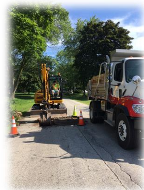
DPW Manhole Rehabilitation
