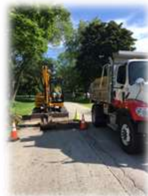
DPW Manhole Rehabilitation
