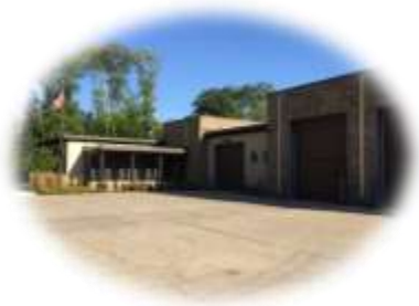
North Shore Fire/Rescue Station #85
