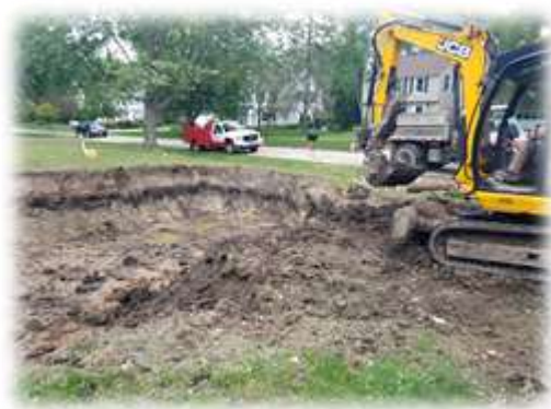
Tennyson Drive Construction
