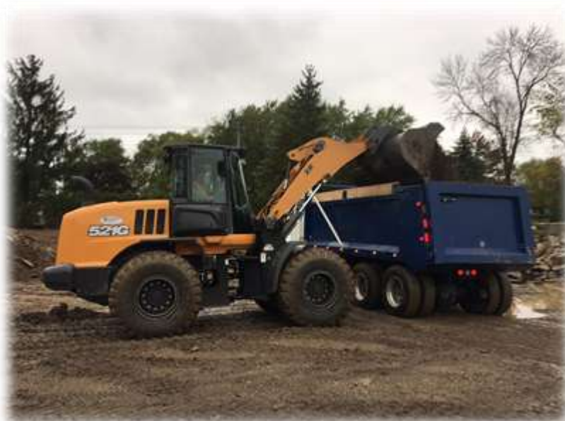
Public Works Yard Clean-up
