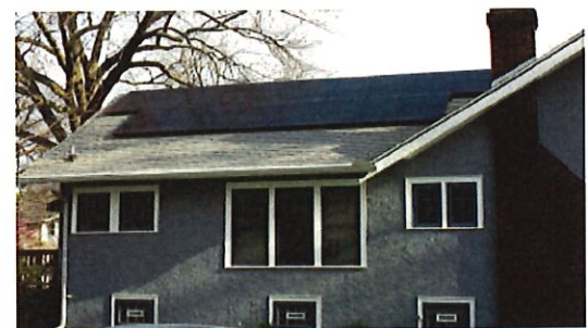
5.10kW array installed on residence as part of Solar Urbana Champaign 2.0 Group Buy.
