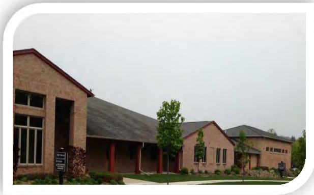
Figure 2 – Village Municipal Building, Regent Road
