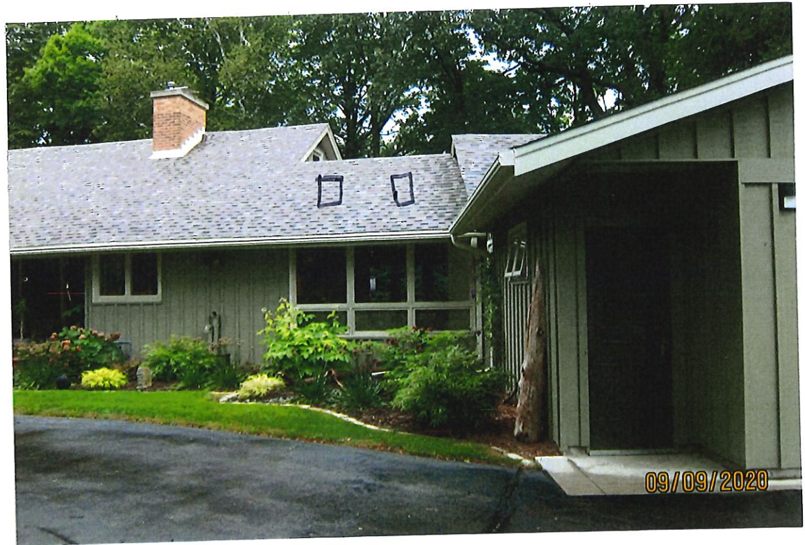
Picture of where skylights will be installed
