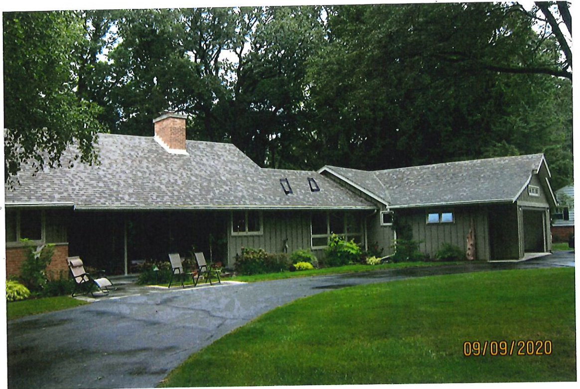
Picture of where skylights will be installed
