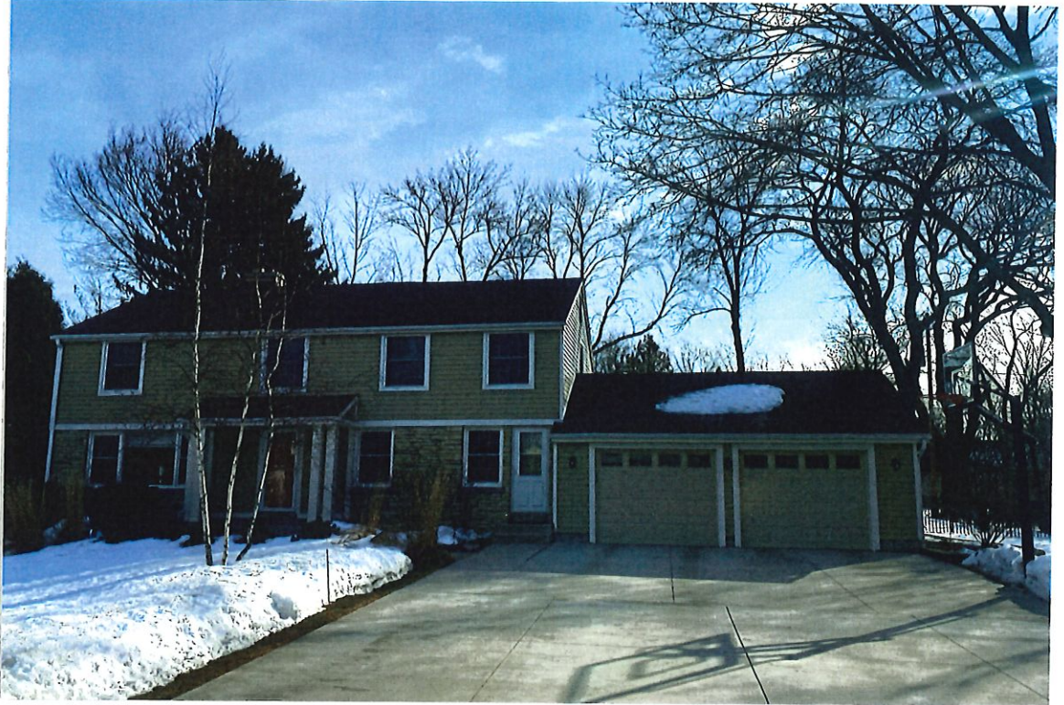
Picture of existing home
