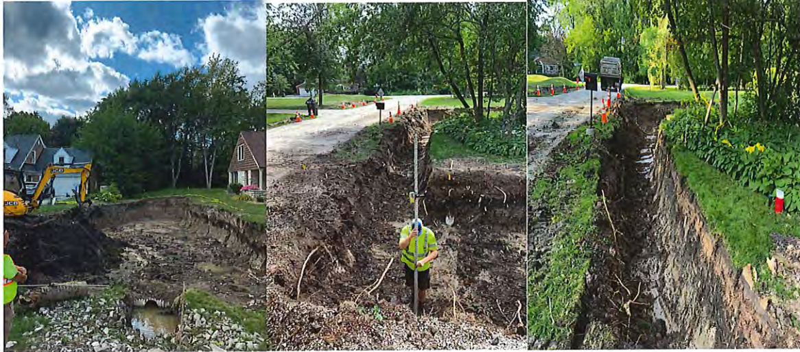
ditch line construction to third bio retention system
