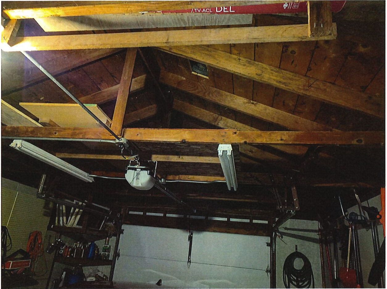
Existing Garage Roof Trusses
