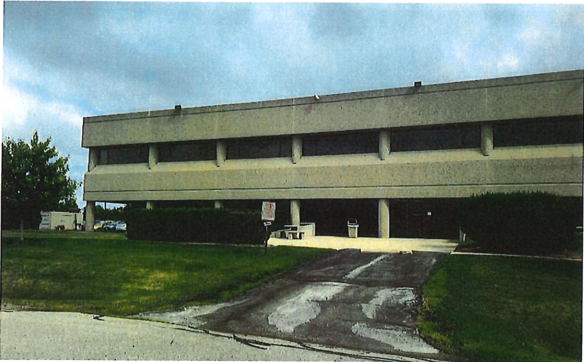
EXISTING SOUTH ENTRY
