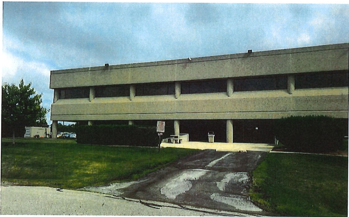
EXISTING SOUTH ENTRY
