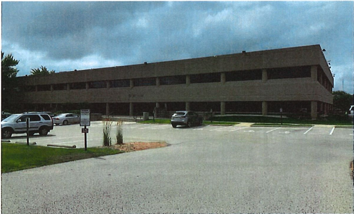
EXISTING EXTERIOR ENTRY
