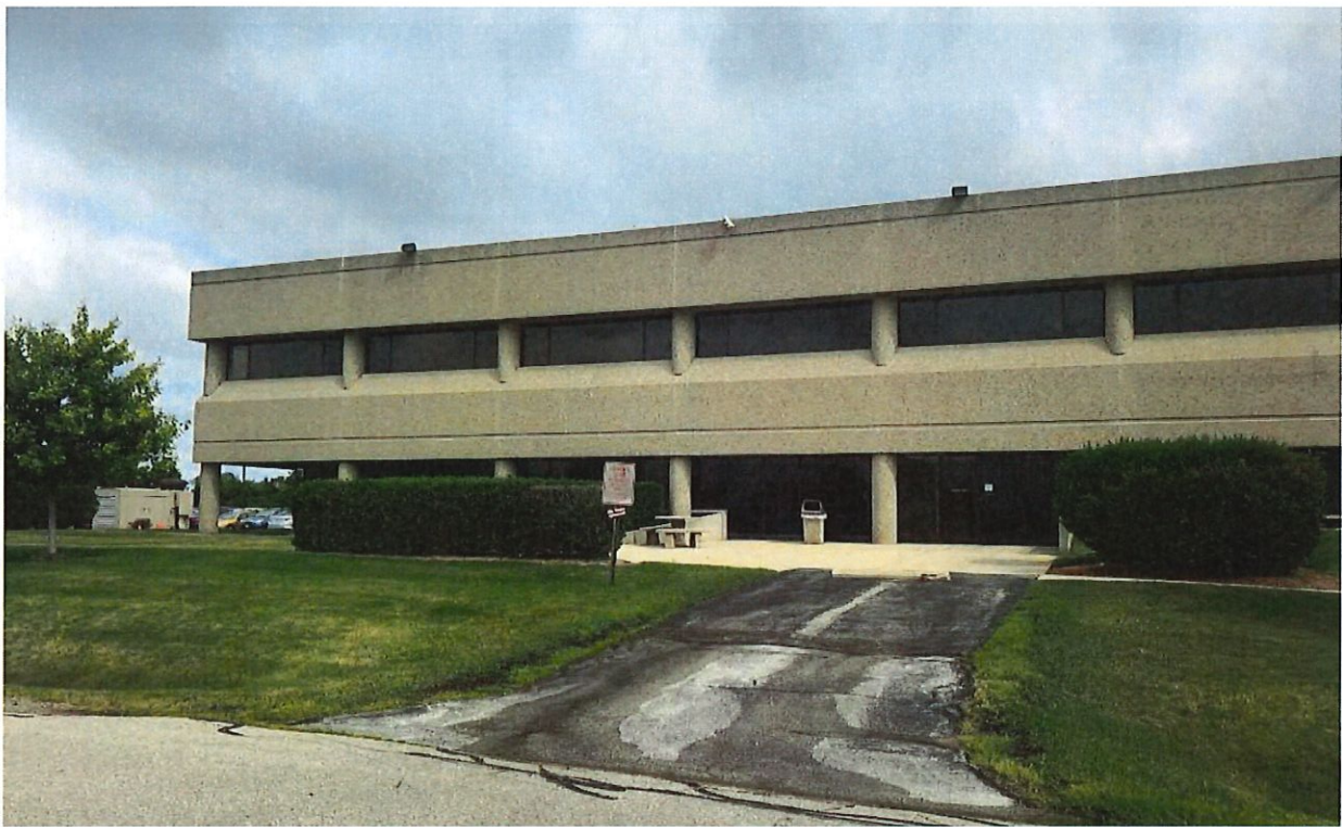
EXISTING SOUTH ENTRY
