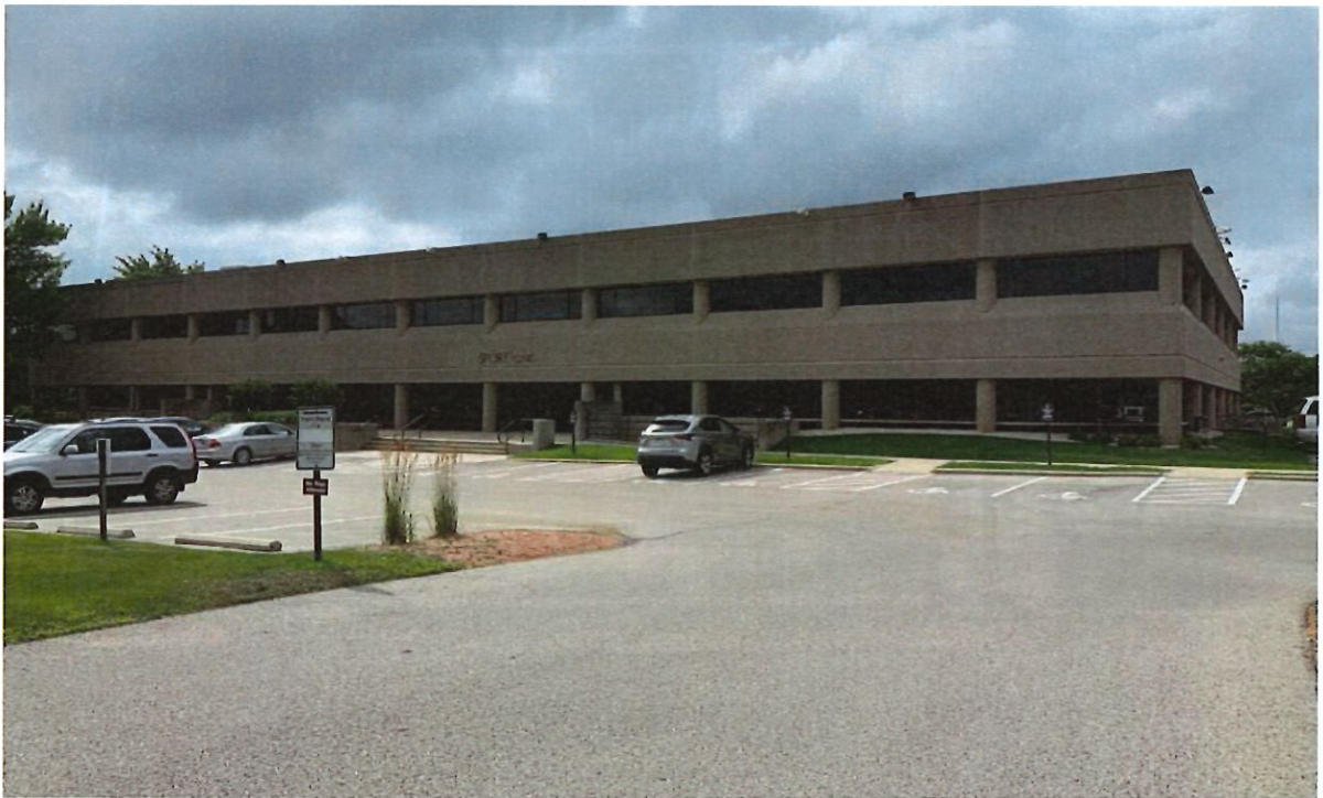
EXISTING EXTERIOR ENTRY
