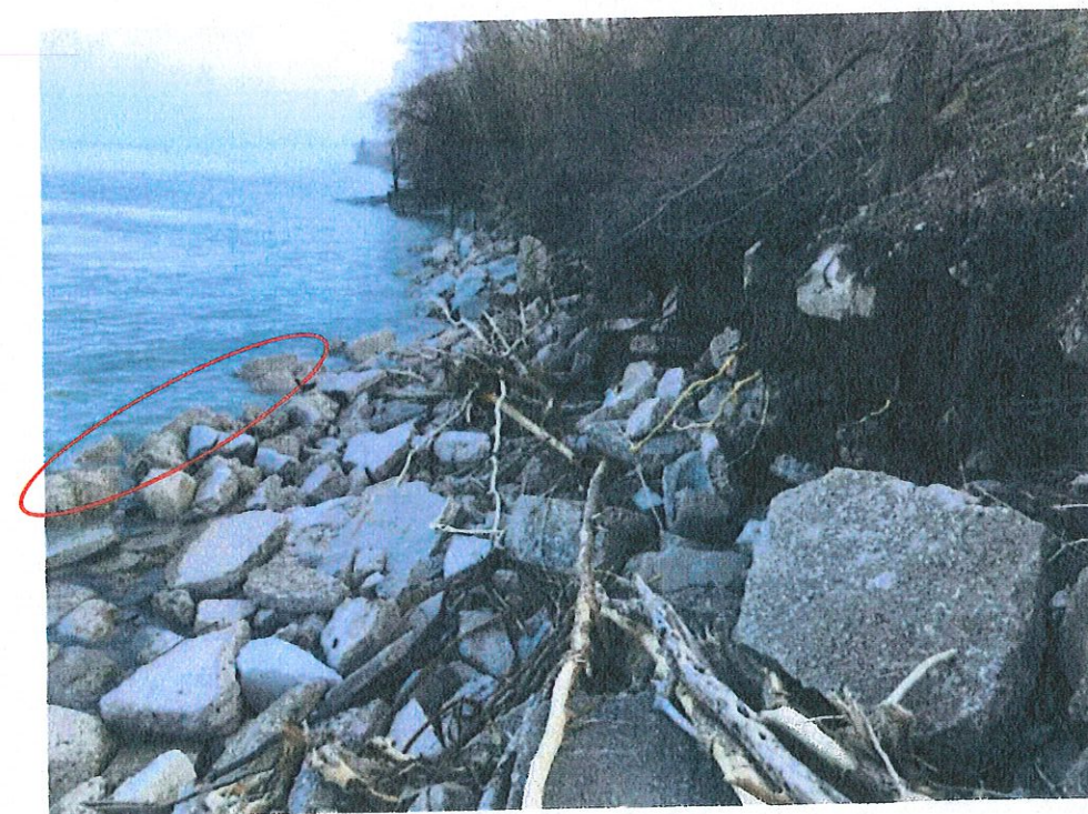
PHOTO 3: LOOKING SOUTH ALONG THE SUBJECT SHORELINE AT THE EXISTING REVETMENT. THE STONES CIRCLED IN RED SHOULD BE SALVAGED AND MOVED WESTWARD.
