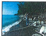
PHOTO 5: LOOKING SOUTH TOWARDS MARTENS PROPERTY AT EXISTING RIP RAP.
