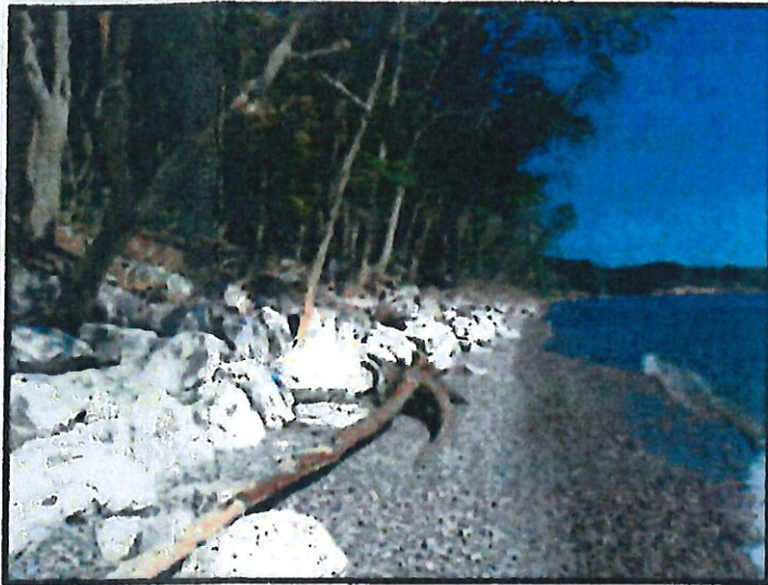
PHOTO 2: LOOKING NORTH AT EXISTING RIP RAP REVETMENT ALONG THE SUBJECT PROPERTY.
