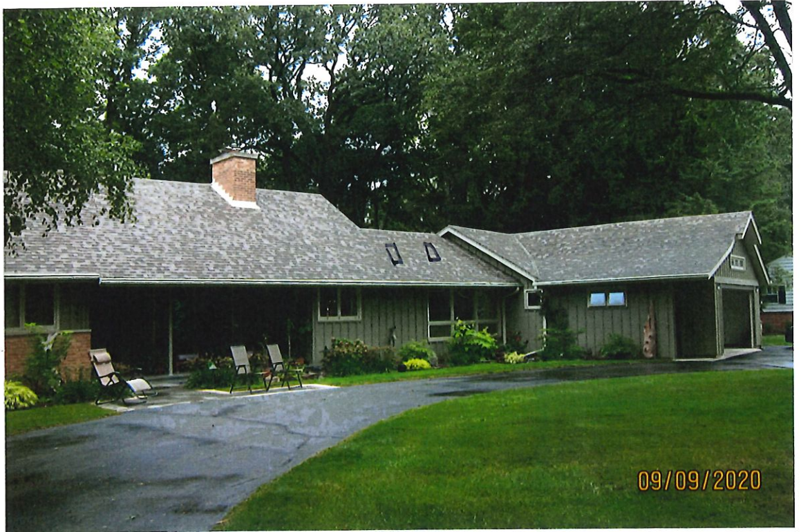
Picture of where skylights will be installed
