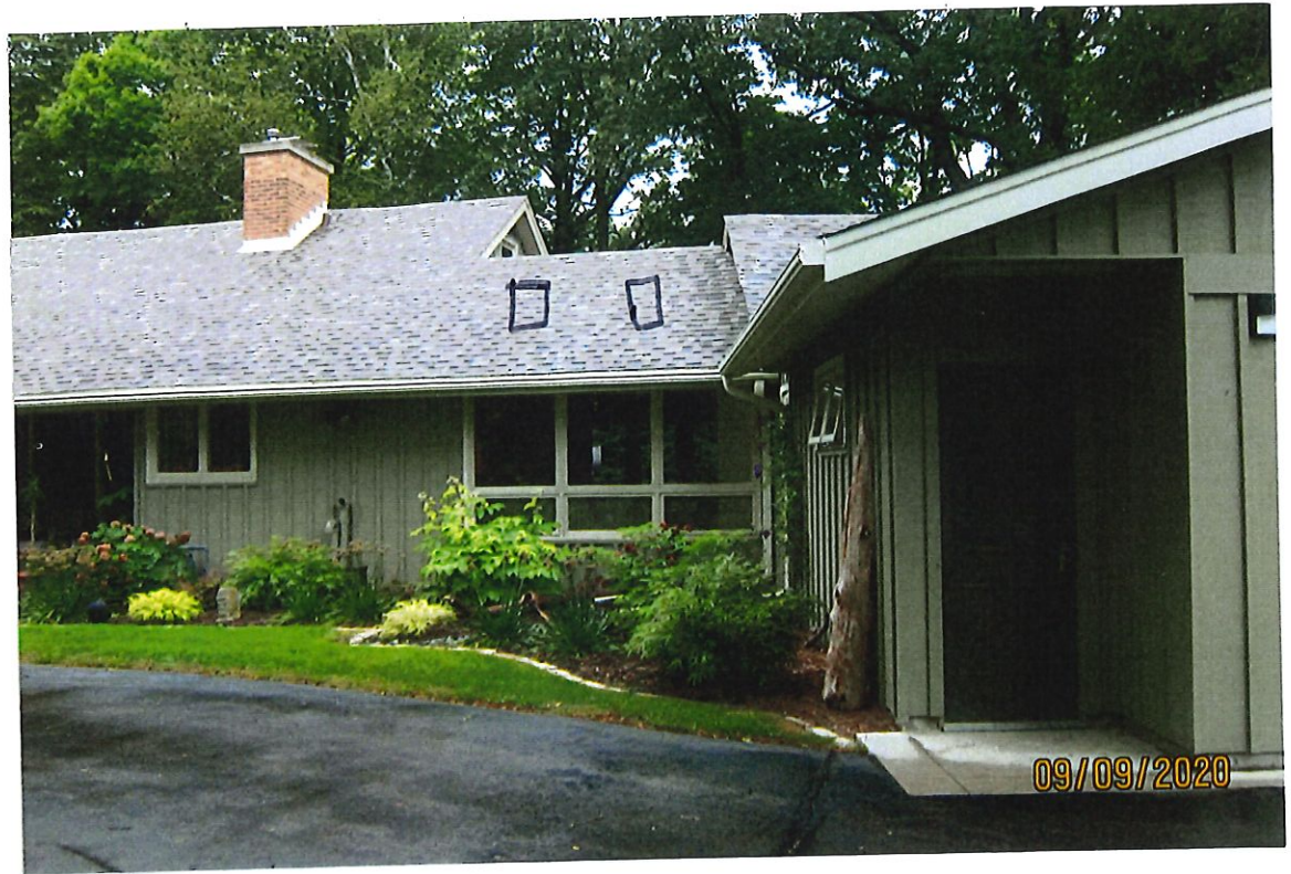
Picture of where skylights will be installed
