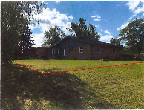
A 1 View From Street: North looking South West NTS
