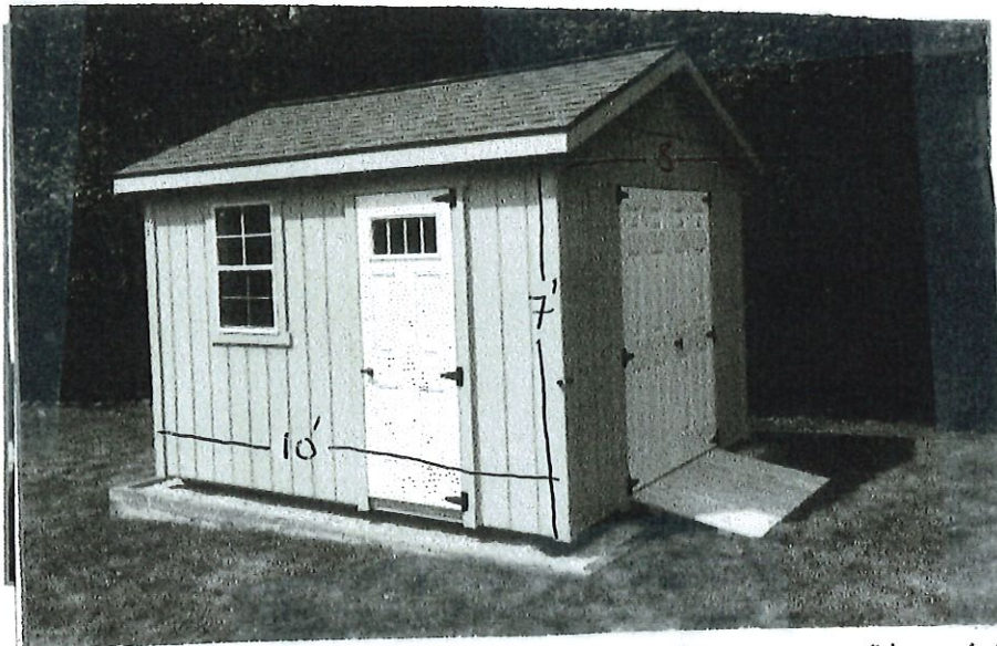
Custom Shed Walls
