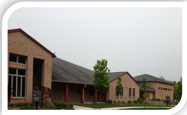
Figure 2 – Village Municipal Building, Regent Road
