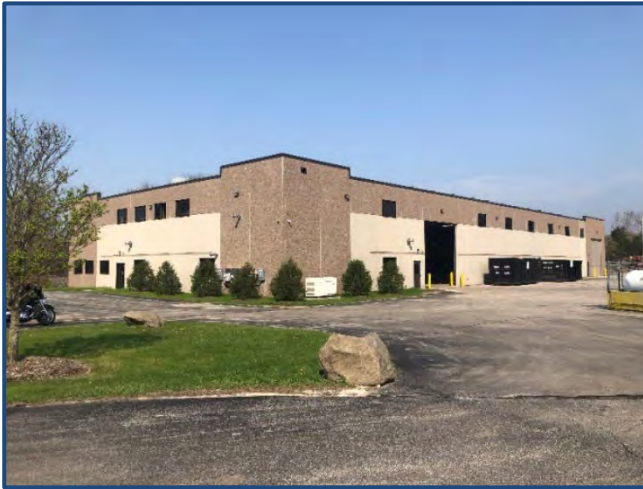
Figure 2. Department of Public Works Facility
