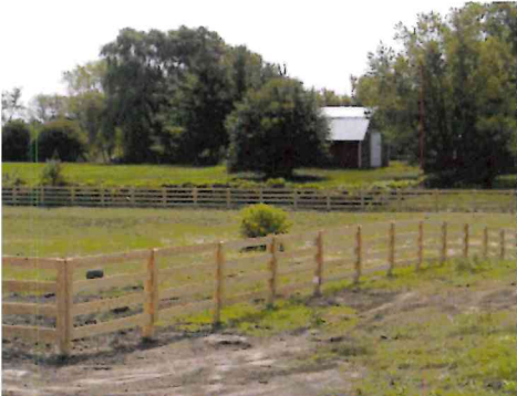
Corral Fence 4 Rail with Cover Board
