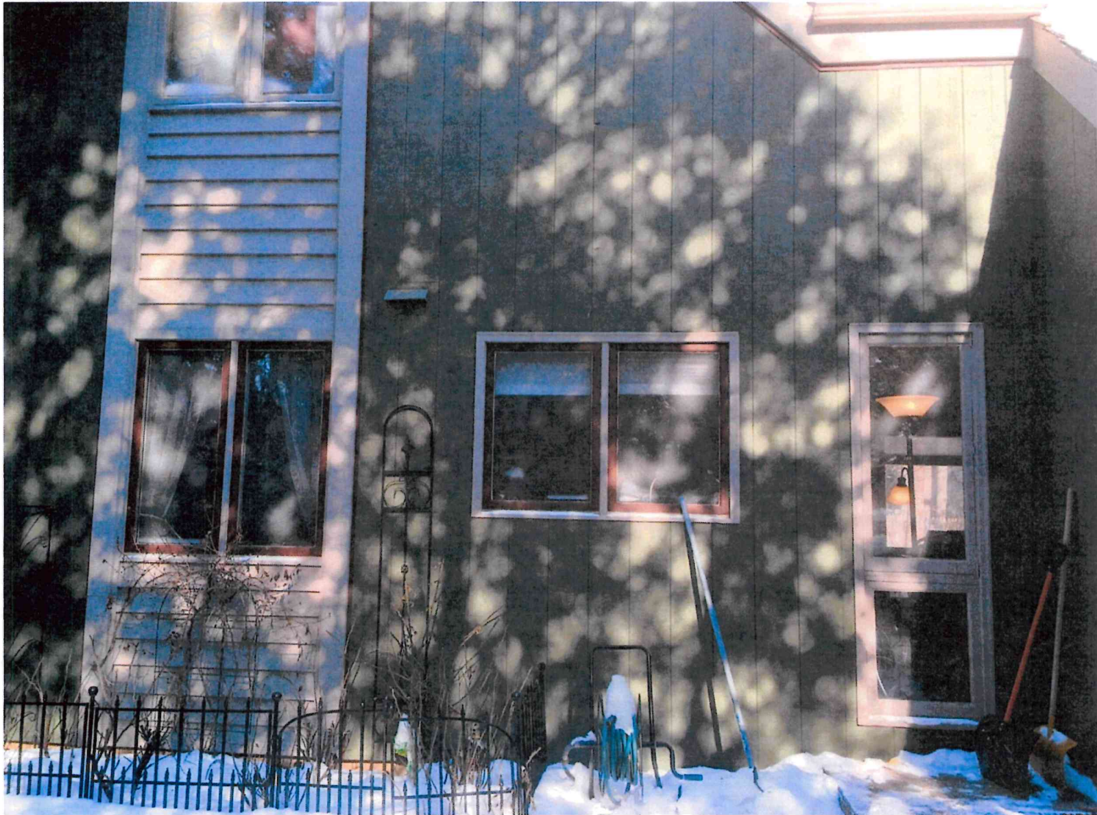
EXISTING - SIDE OF HOME
